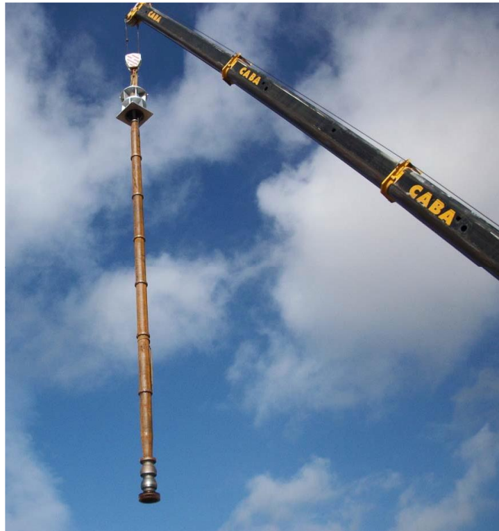
Figure 7-16 Salt Pump in a Commercial Project
